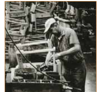
Wood frame assembly 1960s
